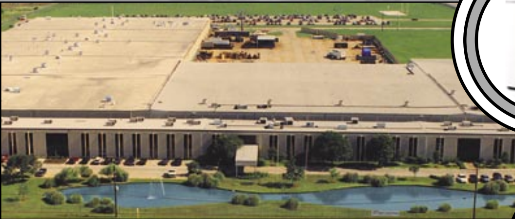
North America Headquarters & Manufacturing Facilities (Houston, TX)
